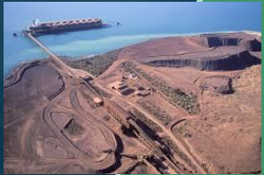
Raw materials access
