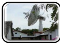
Basi ed infrastrutture operative
